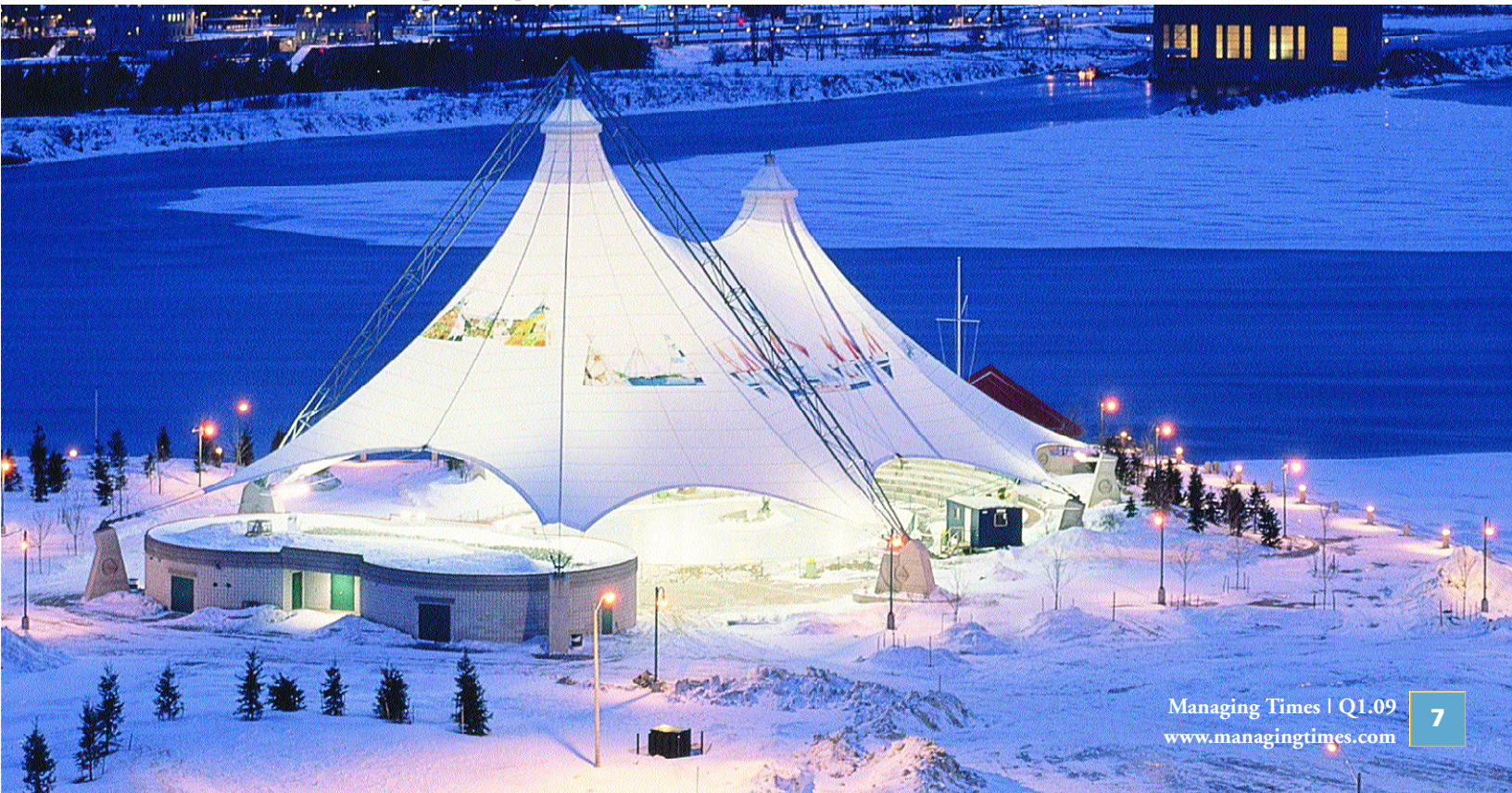
This custom architectural tension structure, part of the Sault Ste. Marie, Ontario, Canada, welcome center, features Shelter-Rite® fabric, coated with Tedlar® PVF film for ease of cleaning and UV protection.
