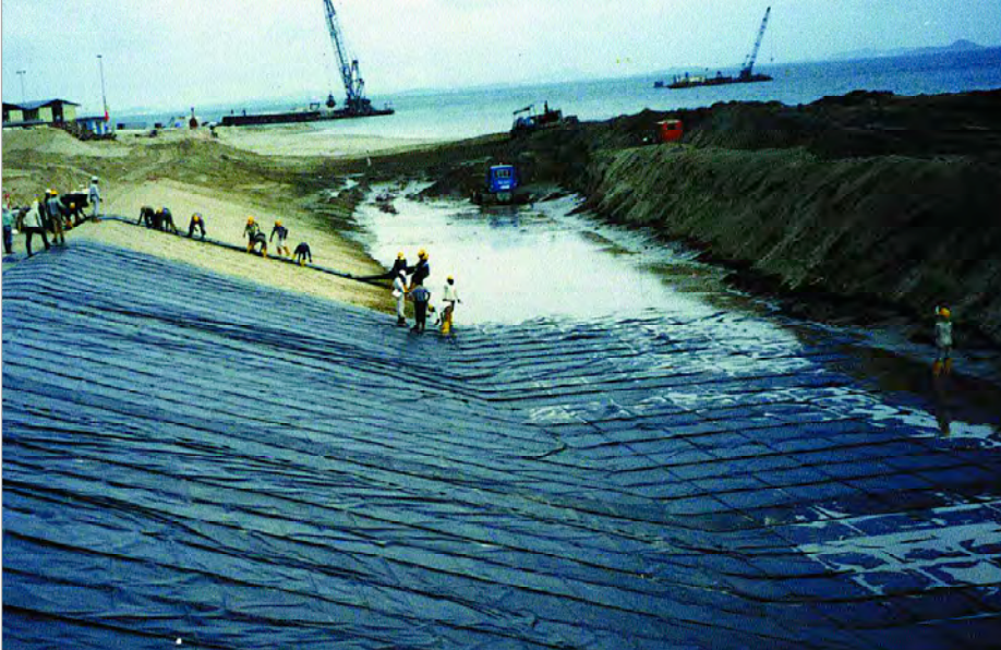
This geomembrane system was used as an alternative to clay-based systems to line an offshore waste-containment bund (embankment or dike) for the government of Singapore.
