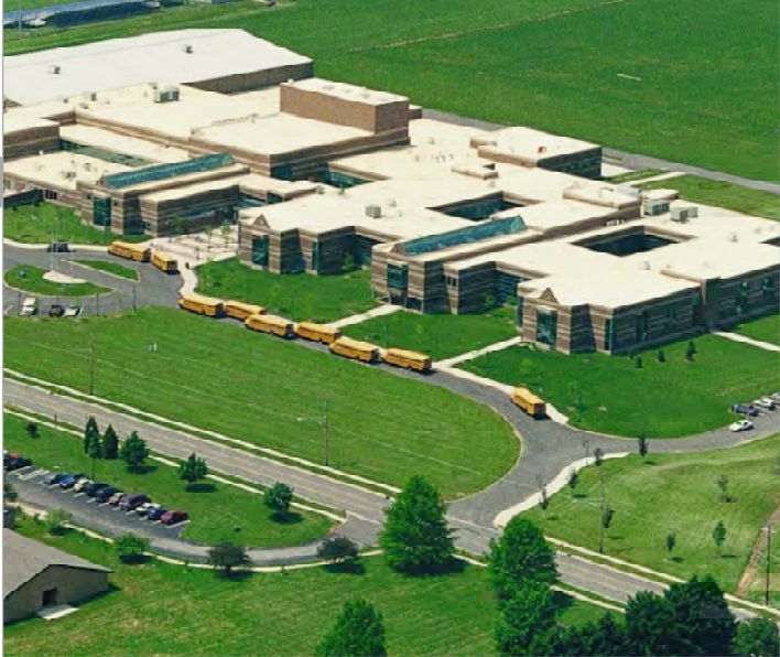
Seaman's Fiber-Tite® roofing system was chosen to cover the new state-of-the-art high school and community center in Wooster, OH.
